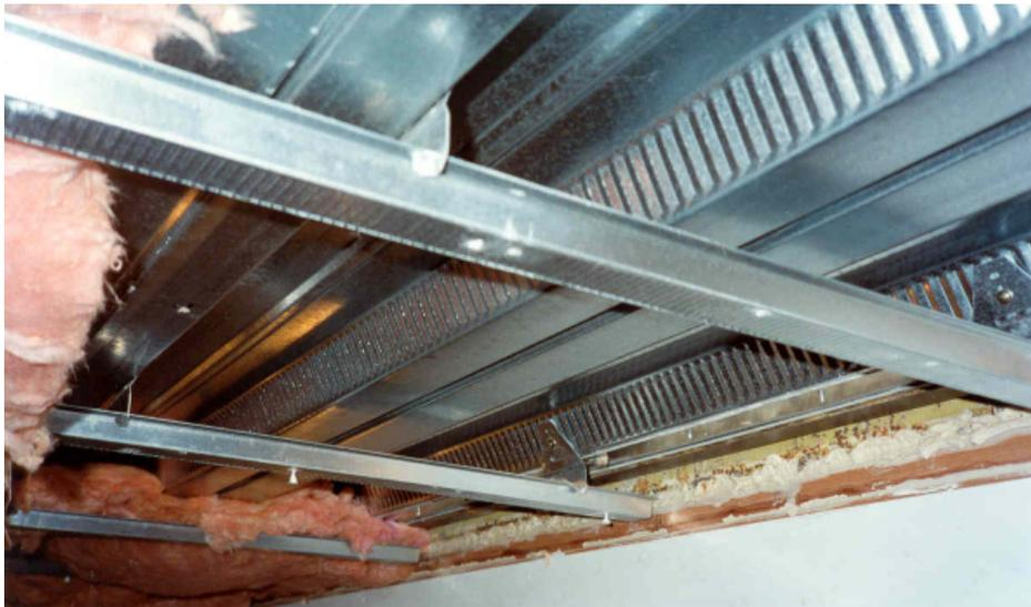
**Figure 1: Underside of floor showing Hibond Steel Decking with USG direct fix clip and steel batten ceiling suspension system.**
