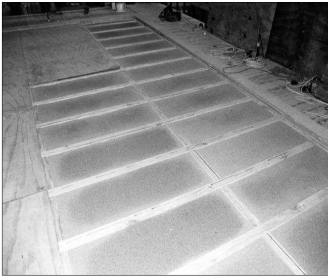
Figure 7: Left: RMS surface velocity for the design with sand-sawdust and sand-only upper layer. Right: Photo of sand-sawdust layer before it is covered by plywood
