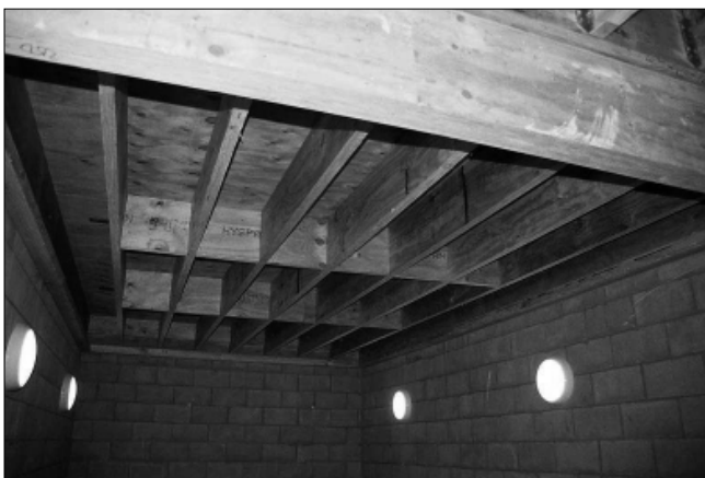
Figure 11: Transverse stiffeners.
