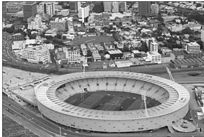
Figure 1: Aerial view of Westpac Stadium.
