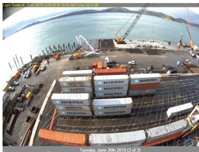
Figure 8: Photograph taken seconds after a 93 dB L_{Amax} trigger event on June 26 at 10:59 am.
