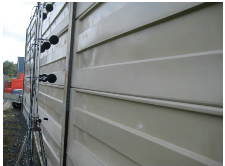
Figure 2: Microphone array in position for in-situ testing
