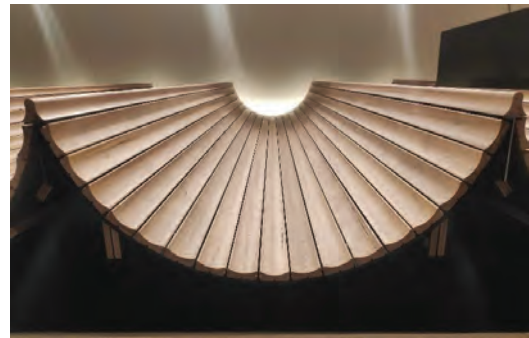
Figure 6. Detail of fluted timber battens
