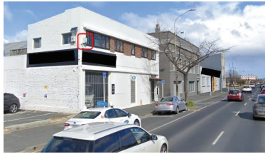
Figure 4: Example of remote access device installation near busy road
